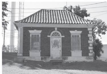
Reservoir Hill Pump House
